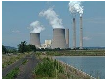
The coal-fired Gavin Power Plant in Cheshire, Ohio
