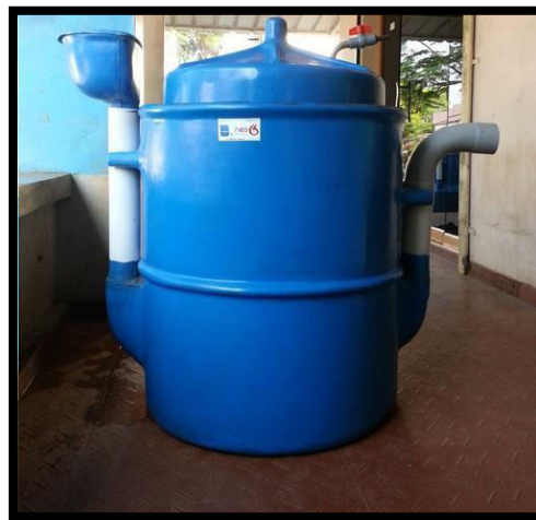
(Fig.4.4 :Small Scale Anaerobic Digestion (Bio-Gas))
