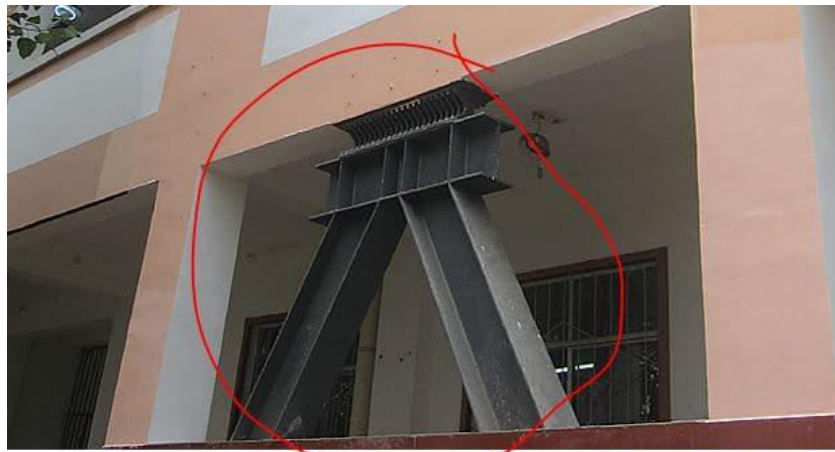
[Fig.1.7: Metallic Yielding Damper Installed in Multistorey Building]
