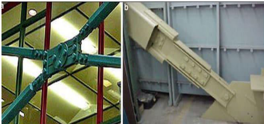
[Fig.1.5: Friction Damper]
