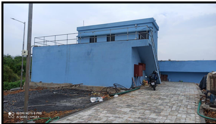
(Fig.5.3: Pump House for inlet Raw Sewage Water)
